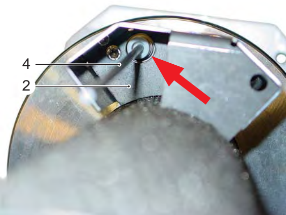
Annular gap at the ionisation electrode
